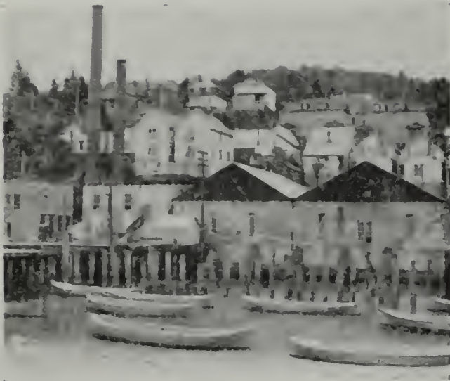
Astor Street Generating Station at Astoria - July, 1910
